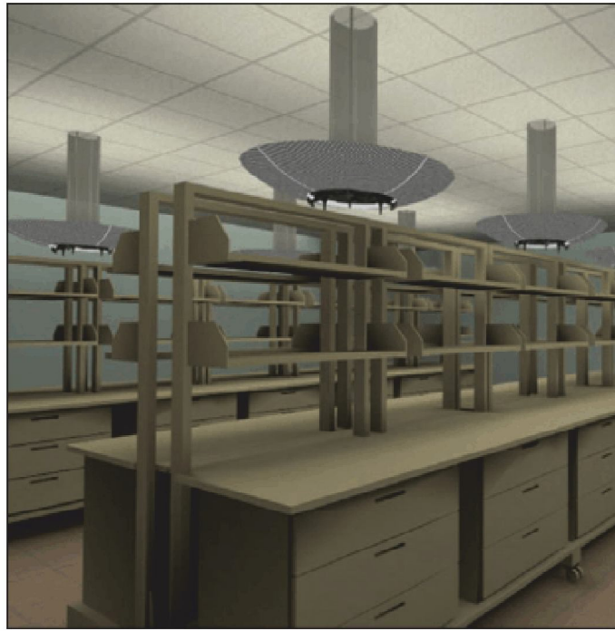
Figure 6: Conceptual study of a lighting array incorporated within the electrical, data, gases overhead service trunk. This scheme provides good lighting for benches located either parallel or perpendicular to the service trunks. Source: Flad Associates and Pivotal Lighting Design/ Affiliated Engineers.
