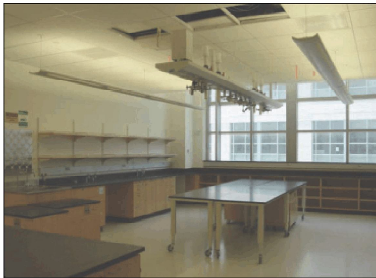
Figure 5: Aisle-mounted indirect luminaires suspended in relation to the overhead service trunk can maintain good-quality lighting regardless of the position of the movable benches, as long as the ceiling remains somewhat consistent.
